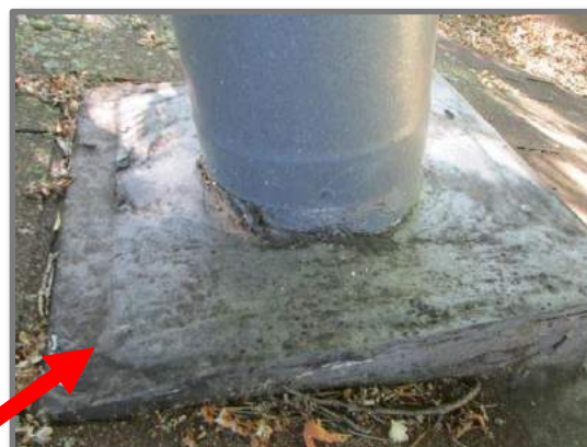
The B vent is rusted inside (left) and tar covered outside on the roof (right)
