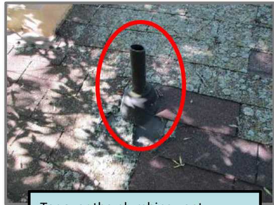
Tar over the plumbing vent (above) and furnace vent (below)
