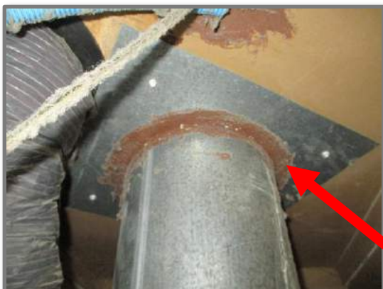
The B vent is rusted inside (left) and tar covered outside on the roof (right)
