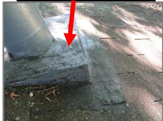
Tar over the plumbing vent (above) and furnace vent (below)
