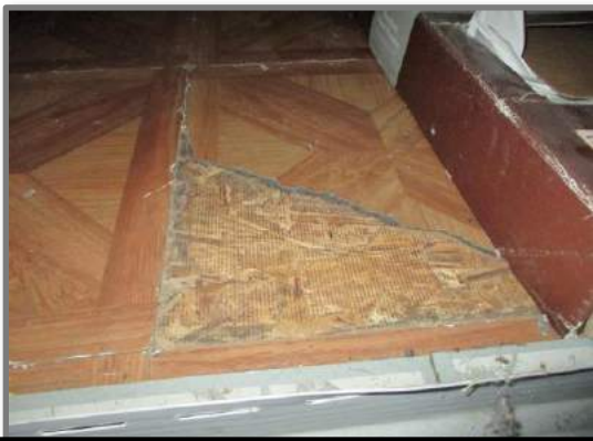
The flooring inside the storage area is whipped
