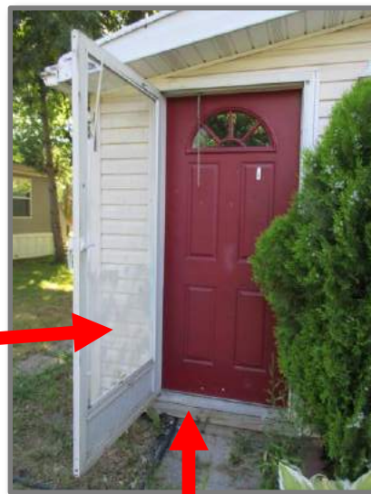
This wood needs paint to protect it from damage
