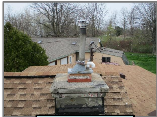
Chimney damage visible
